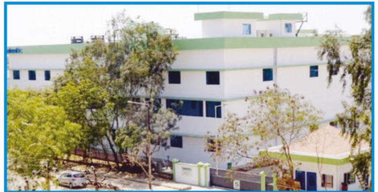
Unit-2: Plot No. 5-B&5-c, Sector III, Kandla Special Economic Zone, Gandhidham - 370230
